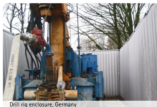
Drill rig enclosure, Germany
