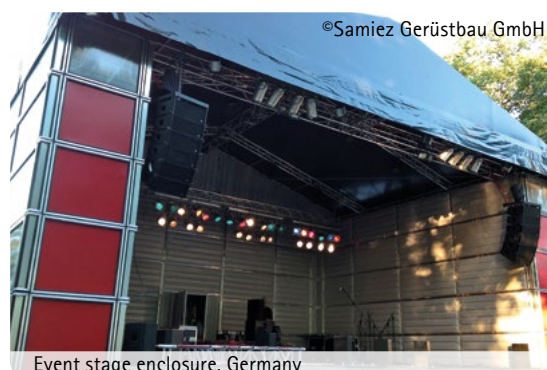
Event stage enclosure, Germany
