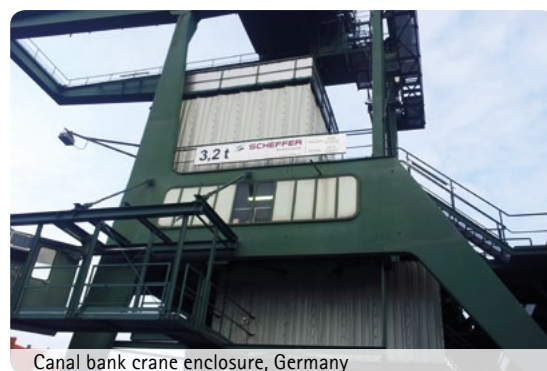
Canal bank crane enclosure, Germany
