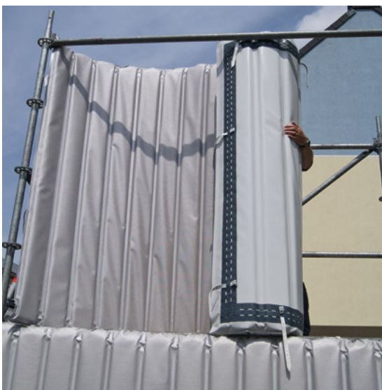
Unrolled in a scaffold section
