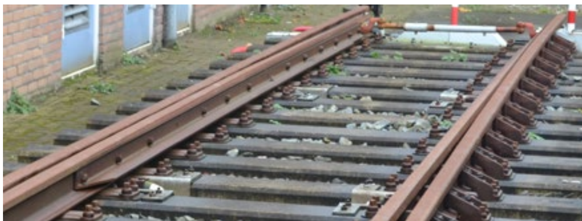
Figure 9: Switch with L-shaped stiffener on the switch rail (switch panel without DeltaSwitch)
