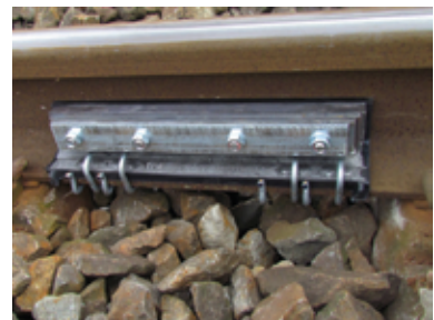
Tuned Dampers assembled on ballast track
