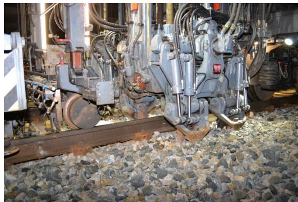
Figure 7. Tamping in a transition zone.
