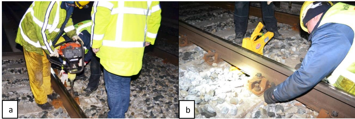
Figure 8. Adjustment of the fasteners.
