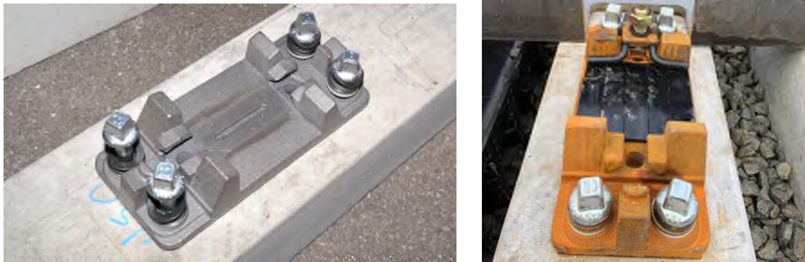
Figure 3 ShimLift, base plate; right picture: including base shim, bolt and clip
