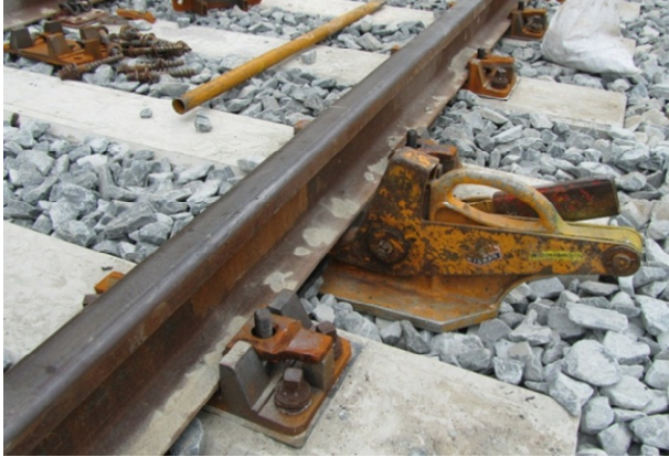
Figure 7 Jacking the rail
