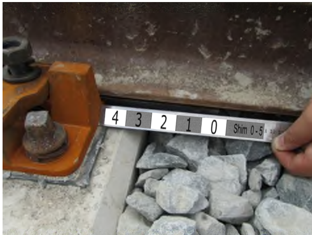
Figure 9 Checking the level of the shim
