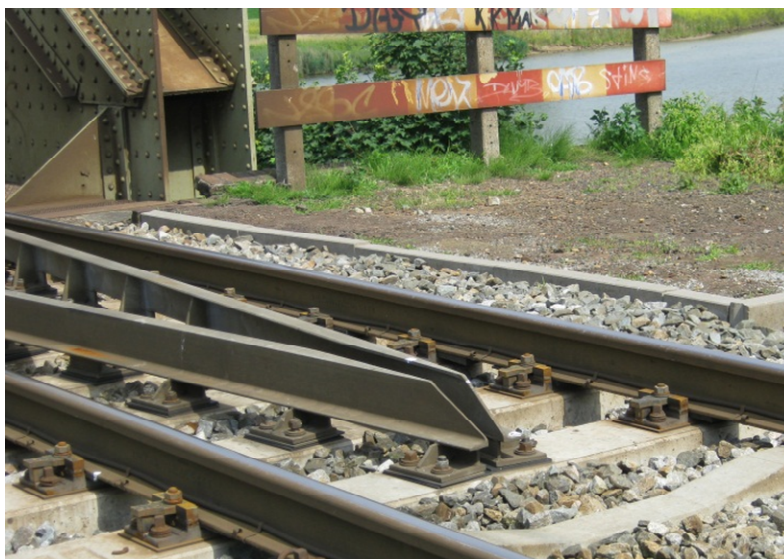
Figure 10 Shimmed derailment provision at transition with ShimLift
