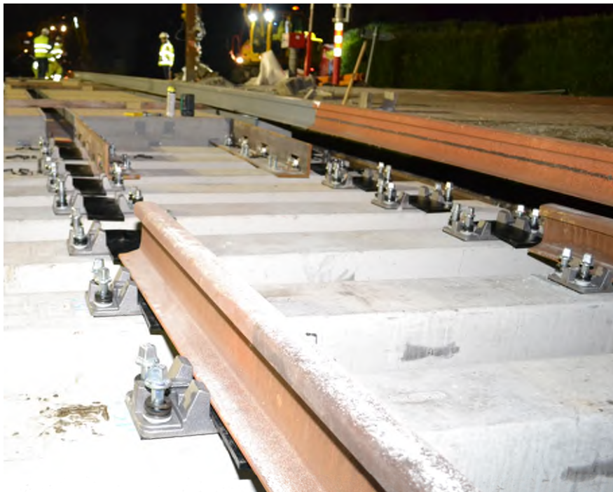
Figure 1 Installation of ShimLift at a transition to a level crossing
